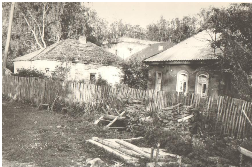
Fig. 1. On the site of this house in the village of Milyukovo, Novoduginsky district, Smolensk region, stood the house where Vasily Dokuchaev was born. Archive of Central Soil Museum (CSM) (Ф. 2. Оп. 39. Д. 4. Л. 28).
